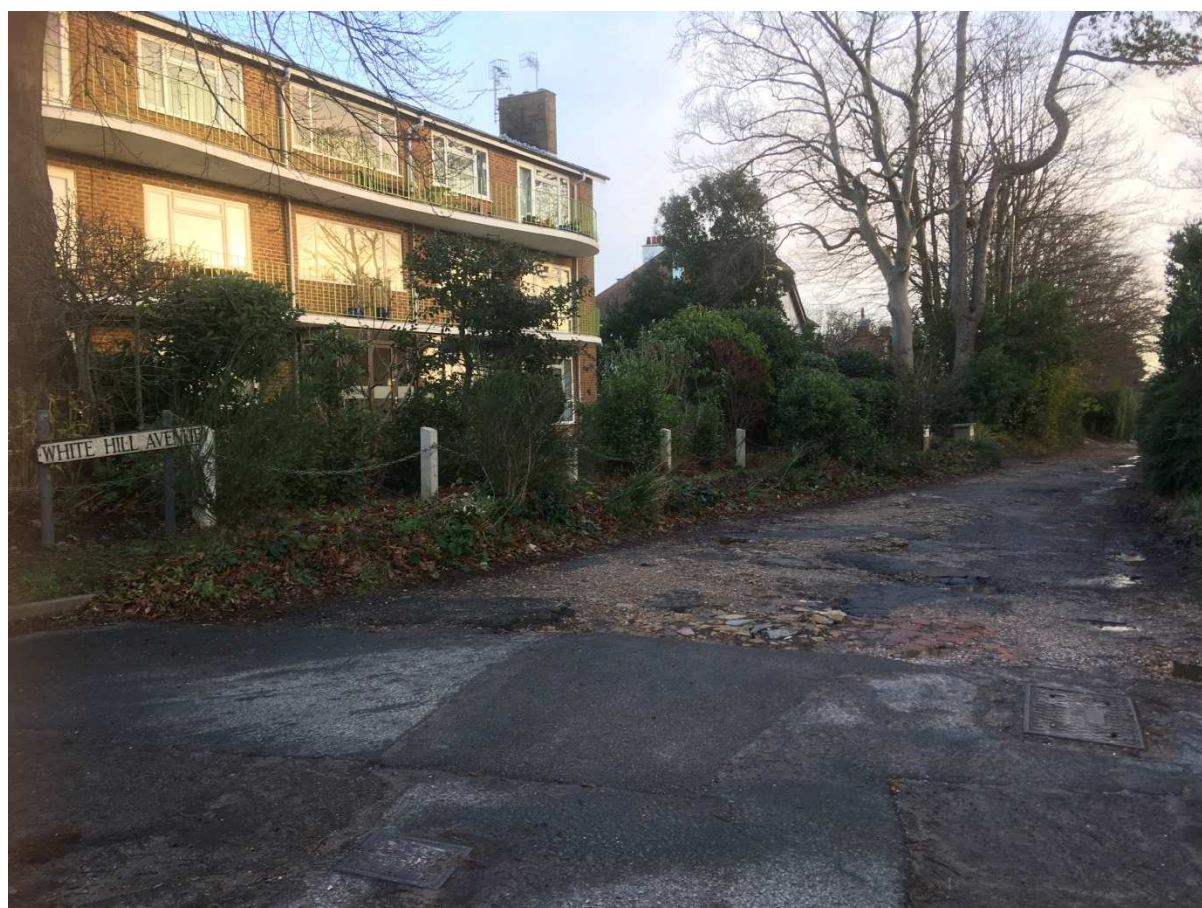
White Hill Avenue not adopted highway- unmade private street
